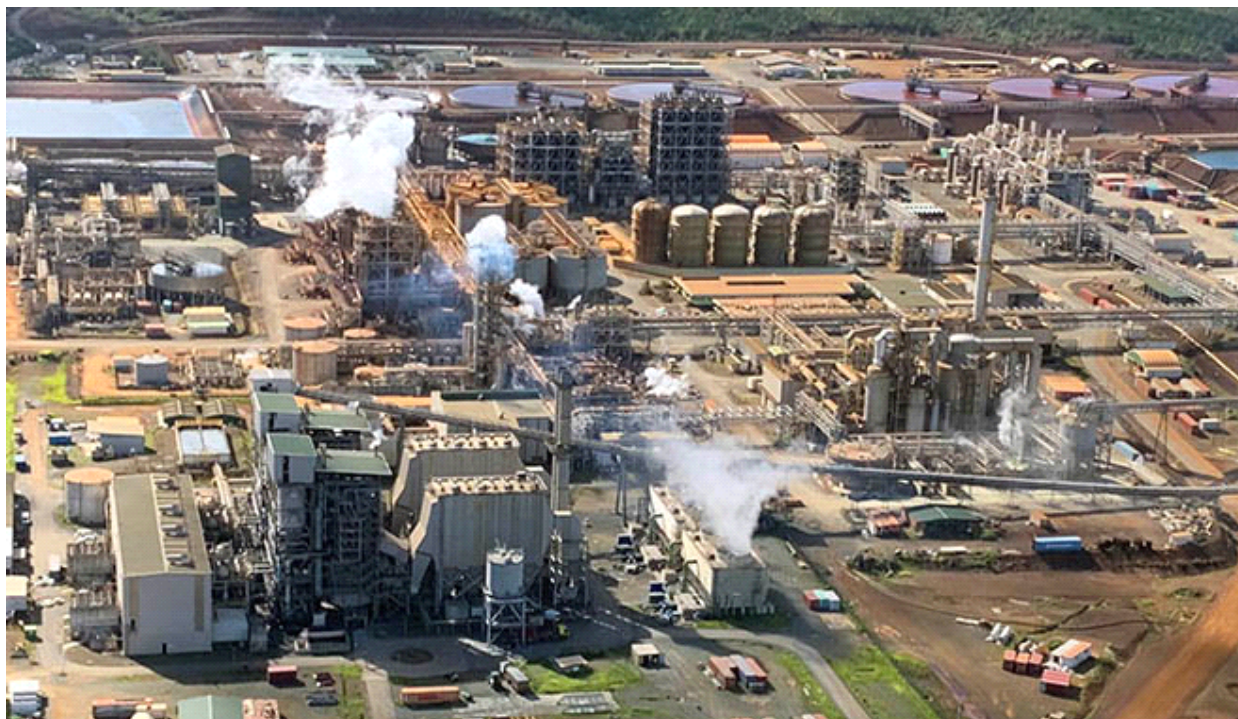
Vale's Goro processing facilities in New Caledonia.
