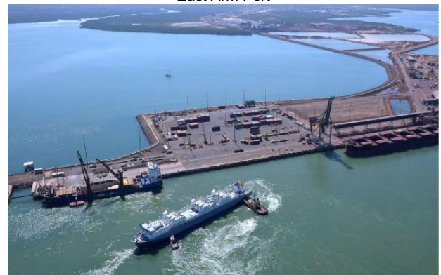
Berth 2 bulk berth (ship docked)
