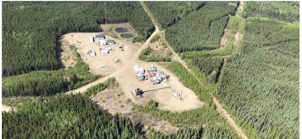
Figure 3.7 – CE1 Tommy Lakes infrastructure - Aerial View
