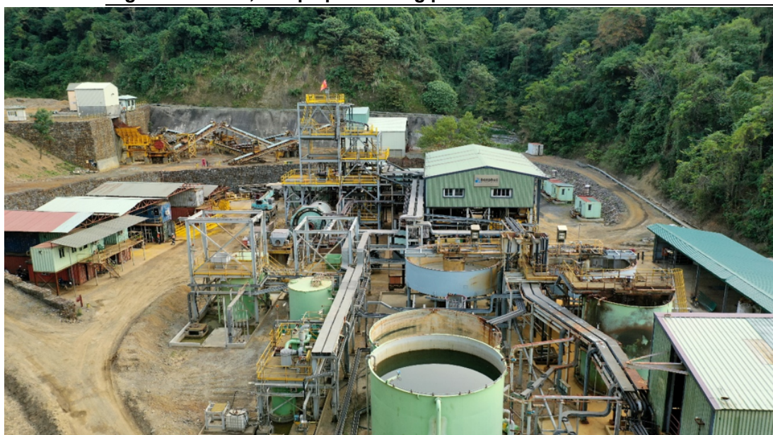
Figure 4.1 – 450,000 tpa processing plant
