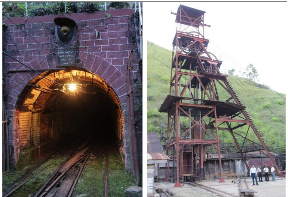
Figure 5.5 – The Tiger Tunnel and the Marmion Shaft headframe
